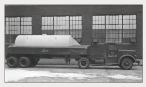
Now Praxair, this photo shows the company's cryogenic tanker in 1949. (Courtesy of Praxair, Inc.)
