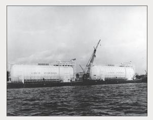
Barges with Liquid Hydrogen for NASA Delivery (Courtesy of: Air Products and Chemicals, Inc.)
