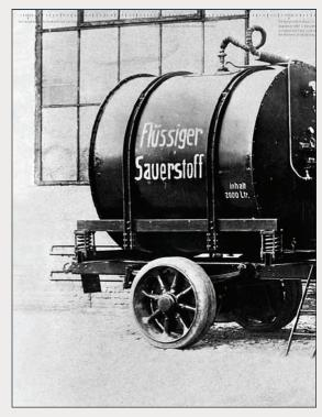
First Portable Tank for Liquid Oxygen (Courtesy of: Linde North America, Inc.)
