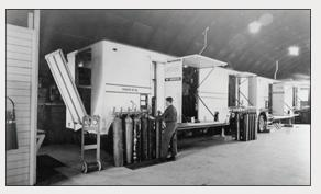
Mobile Oxygen Generators Used by the U.S. Navy to Fill Cylinders (*Courtesy of: Air Products and Chemicals, Inc.*)
