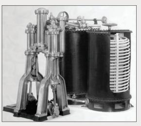
First Refrigeration Machine with Methyl Ether as the Refrigerant (*Courtesy of: Linde North America, Inc.*)
